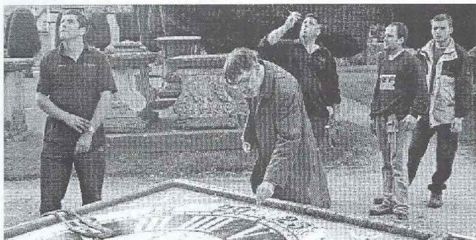
Top, the face is moved and attached to the sling, then lowered diagonally through the scaffolding. Once down, Dr Peters, the diocesan surveyor, examines the gold leaf and the wet rot damage to woodwork
