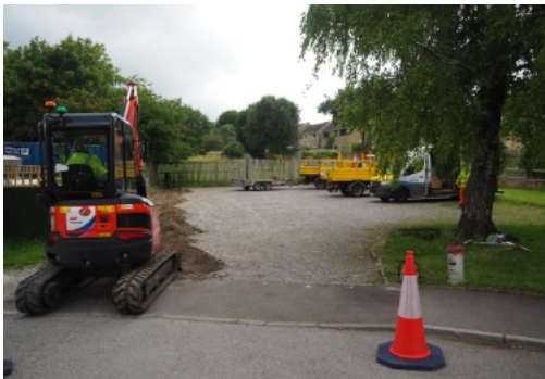
Clearance works underway
